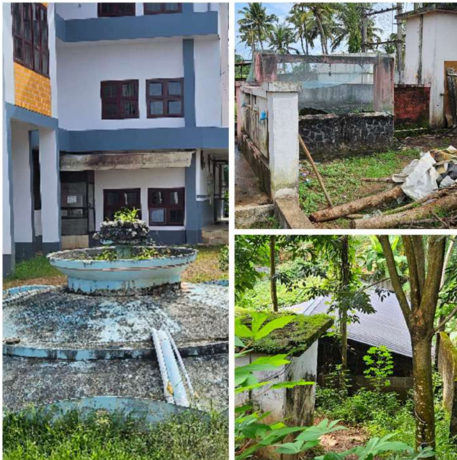
1. Rain water harvesting tank; 2. Open well; 3. Well-maintained pond
