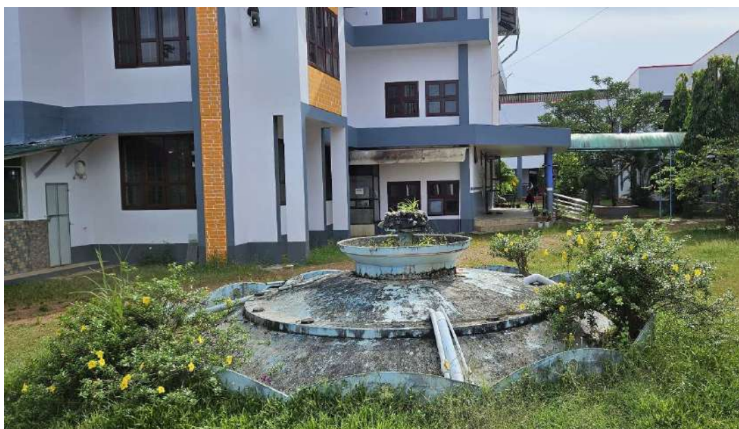
Rainwater harvesting tank of capacity 1.5 lakh Liters
